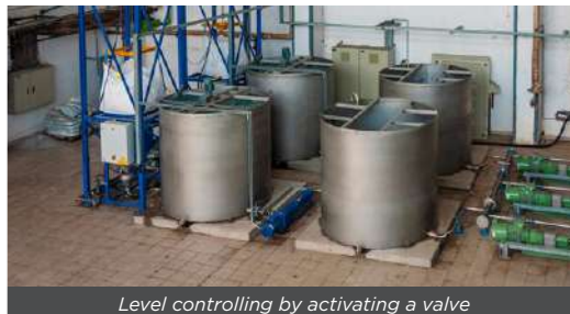
Level controlling by activating a valve
