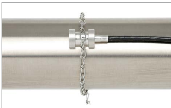
PT100 transducer fixed to pipe
